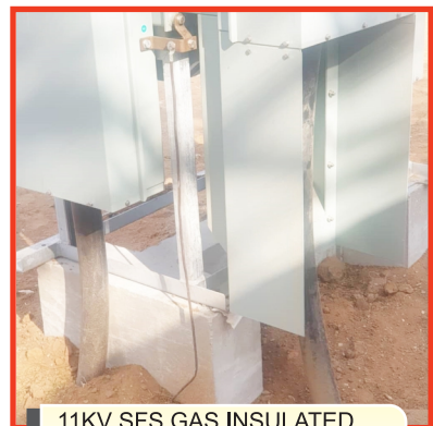
11KV SFS GAS INSULATED RMU INSTALLED
