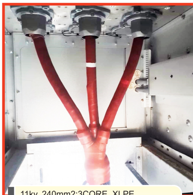
11kv, 240mm 2 ;3CORE XLPE CABLE TERMINATION BOTTOM ENTRY
