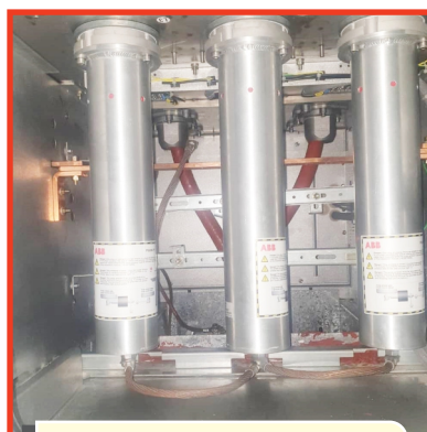
11KV PANEL LIGHTING ARRESTERS, BOTTOM ENTRY
