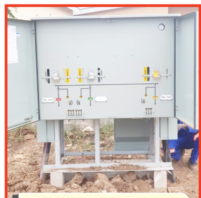
NEW SF6 RMU INSTALLATION COMMISSIONING IN PROGRESS
